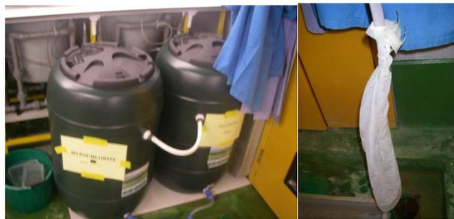
**Figure 2- Water butts used for disinfection of waste water and fine mesh sock on outflow.**
