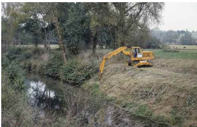
Flail cutting of a river bank in the town of Dropt (Gironde department).
