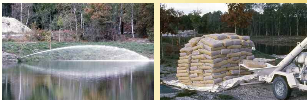
Sediment treatment in a water body by projecting chalk powder mixed with water.
