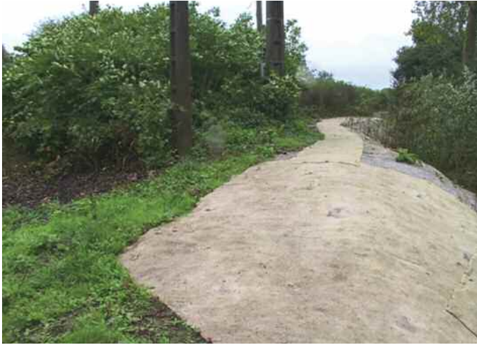
Installation of tarps and willow cuttings in an effort to manage knotweed.
