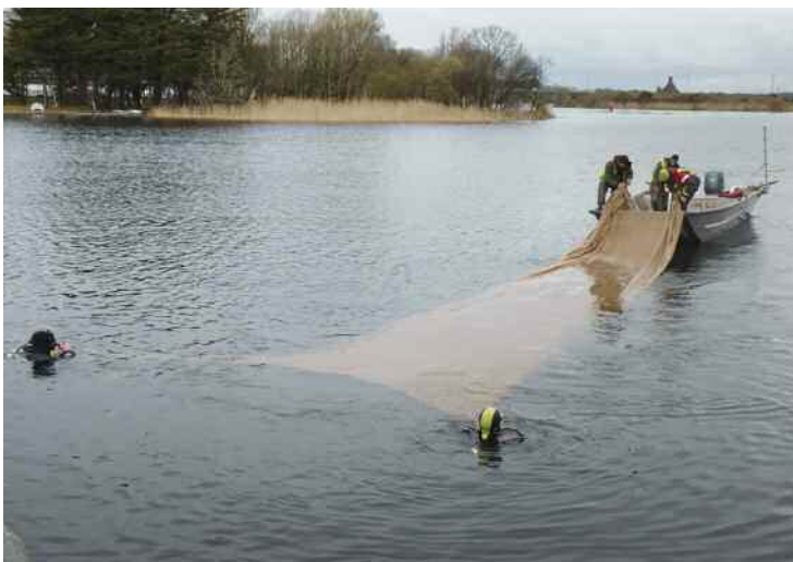
Installing a biodegradable geotextile in Lough Corrib (Ireland).
