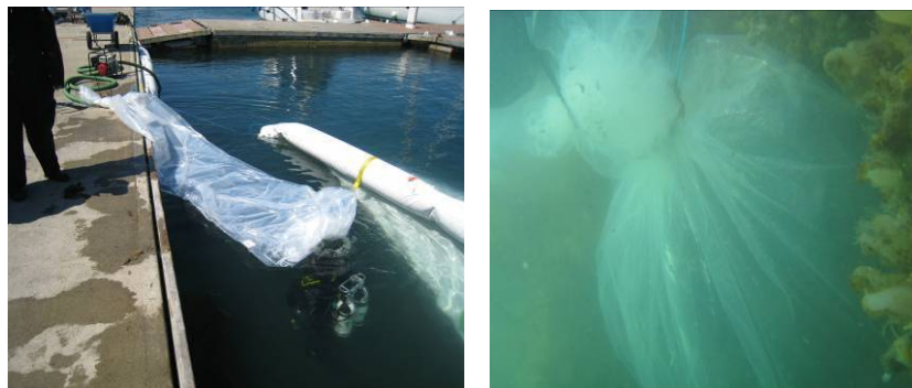
Figure 24 Diver deployment of space filler.
