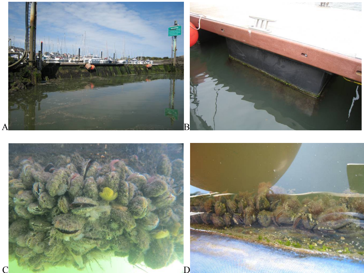
Figure 40 A, Tidal sill at Conway marina; B, Fouling biota at Victoria Dock, Caernarfon; C, Fouling biota at Neyland marina; D, Fouling biota at Conwy marina
