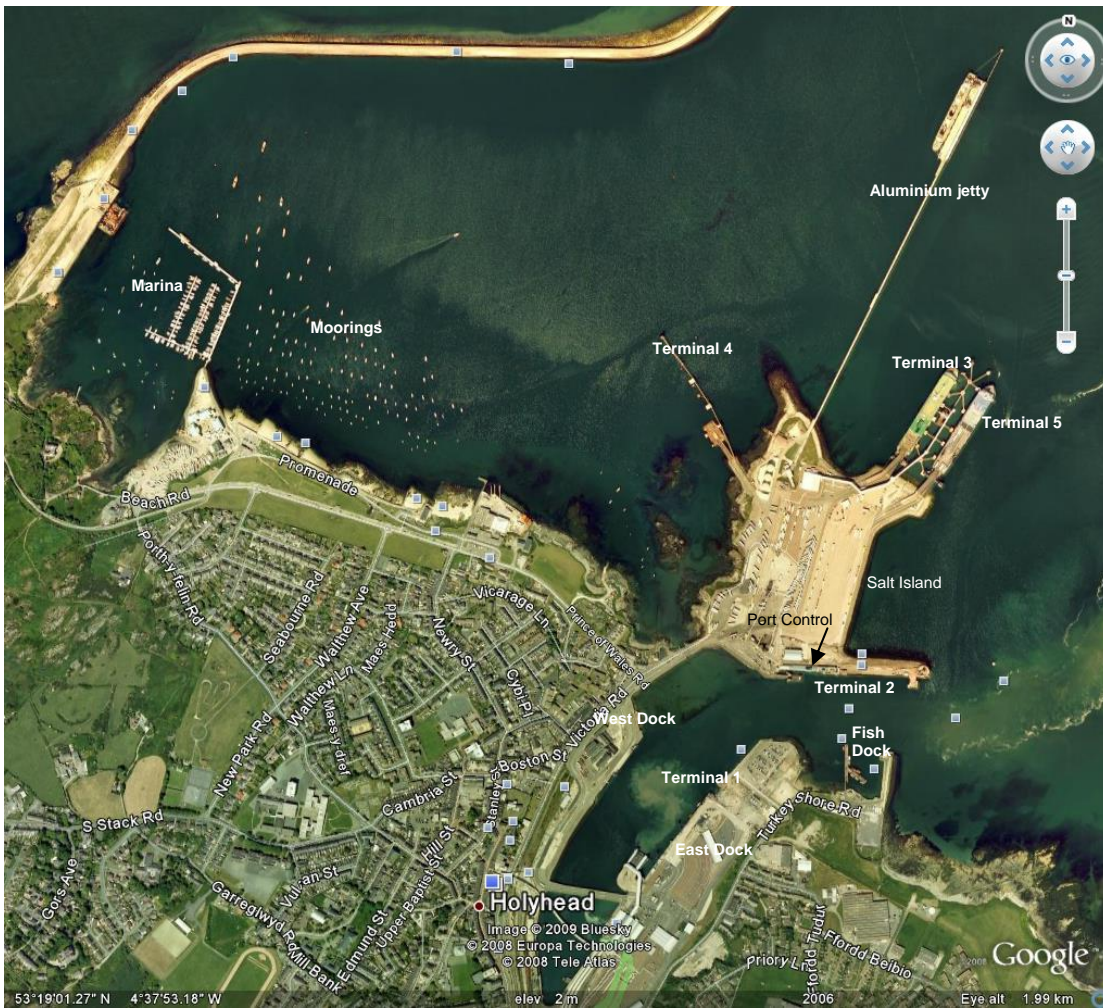
Annotated Google aerial view of Holyhead Harbour showing location of shipping terminals, moorings and marina.
