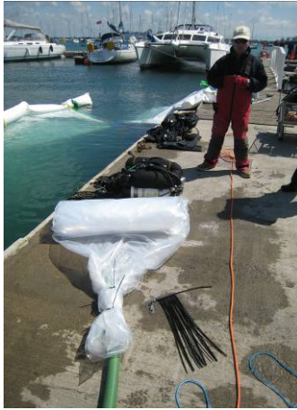
Figure 23 Spacer deployment method. The rolled up bag attached to the water pump outlet on the surface
