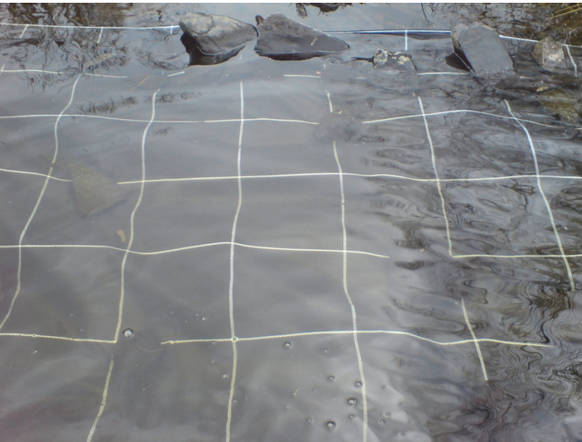
Plate 8. Boulder placement and folded edge of WCF
