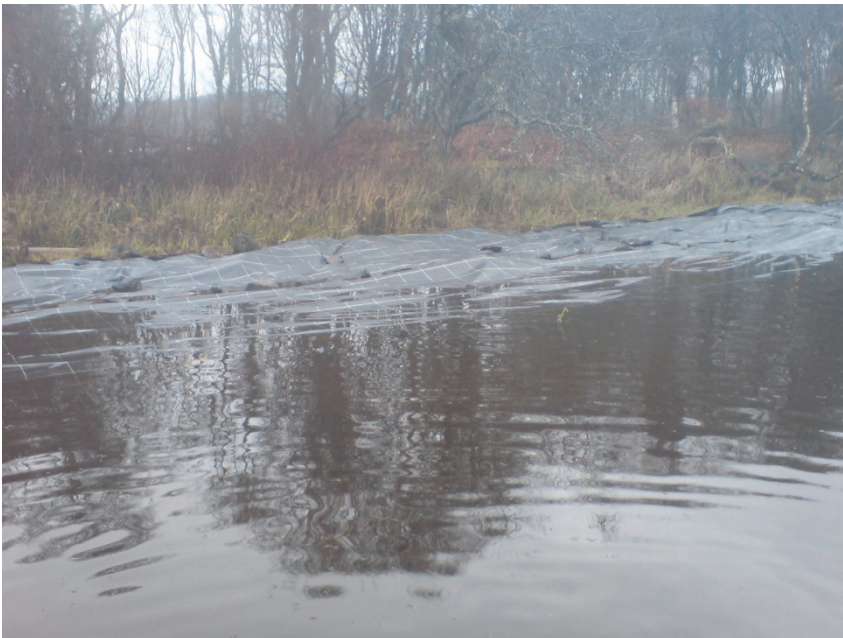
Plate 2. WCF installed at the bay adjacent to Park Hill
