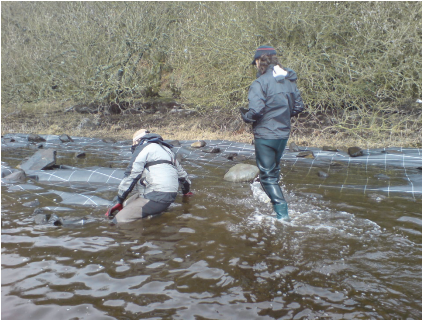
Plate 1. Installation of WCF at Drumwalt Plantation/Scar Islands
