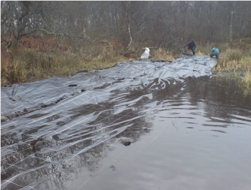
Plate 3. Installation of WCF at Heathery Ward Wood, south bay
