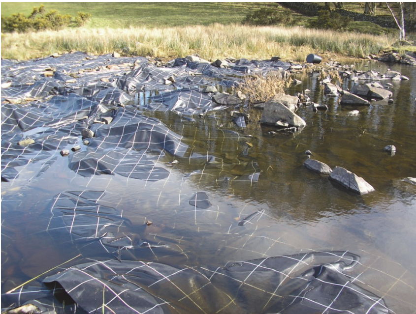
Plate 4. WCF installed over Wee Hill Cove strand line
