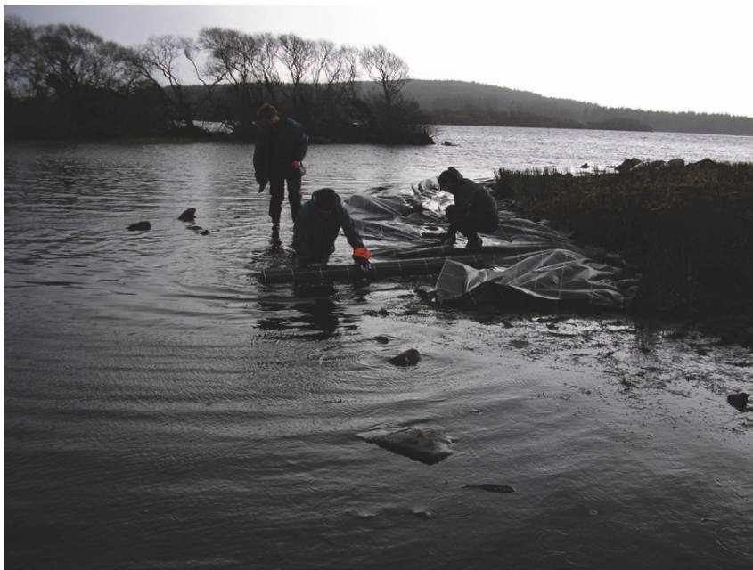
Plate 6. Installation of WCF on west shore, opposite Rowan Island
