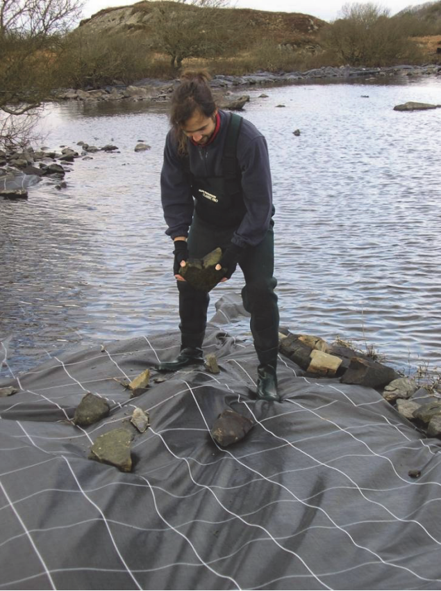
Plate 7. Rock placement at bay on west shore north of Rowan Island
