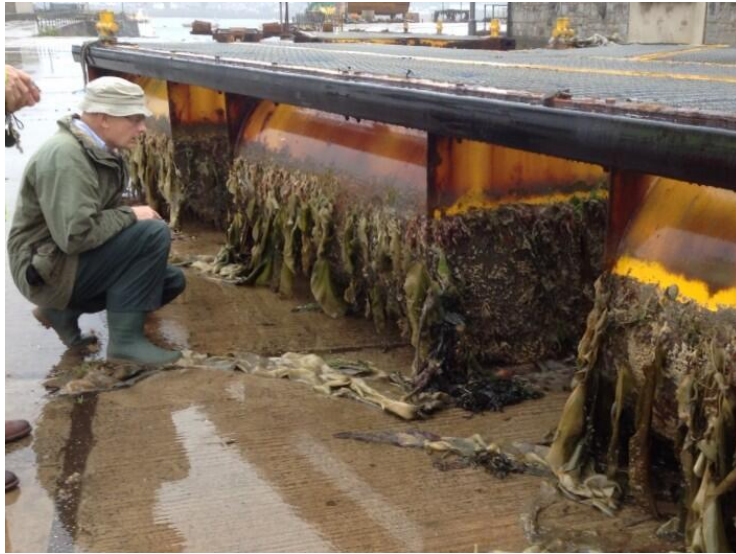
Figure 9: Examining pontoon at Pembroke Dock
